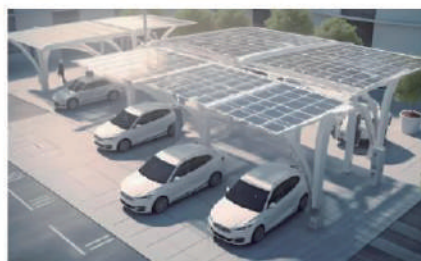
Photovoltaic carport power station
